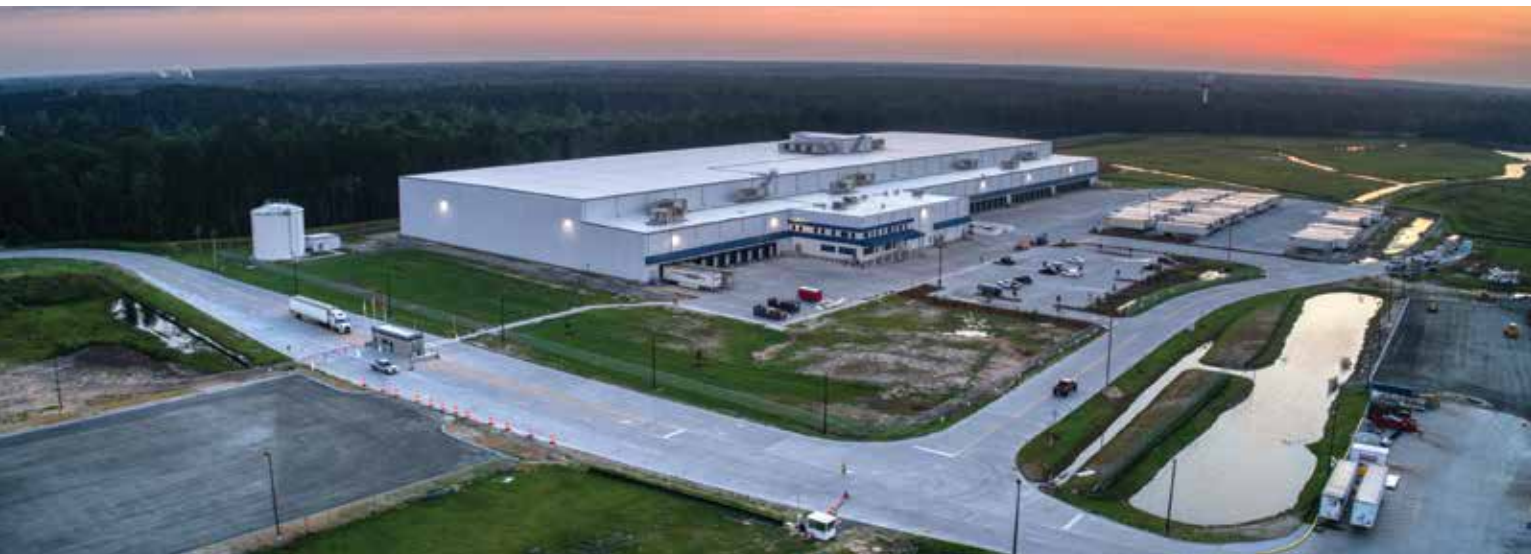
Because of the area's high groundwater, gravel was laid and water continuously pumped offsite to stabilize the ground for construction activities. (Photo courtesy of Primus Builders.)
