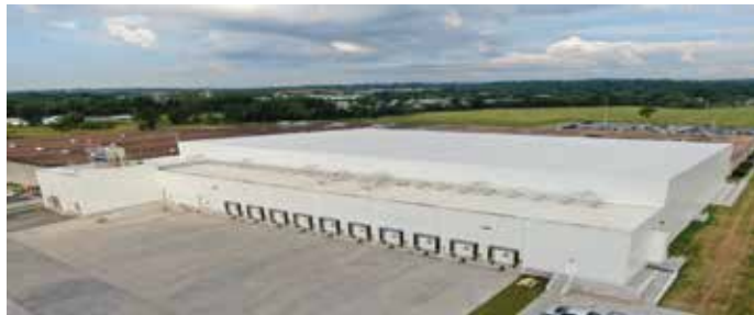
Winchester Cold Storage, Winchester, Virginia
